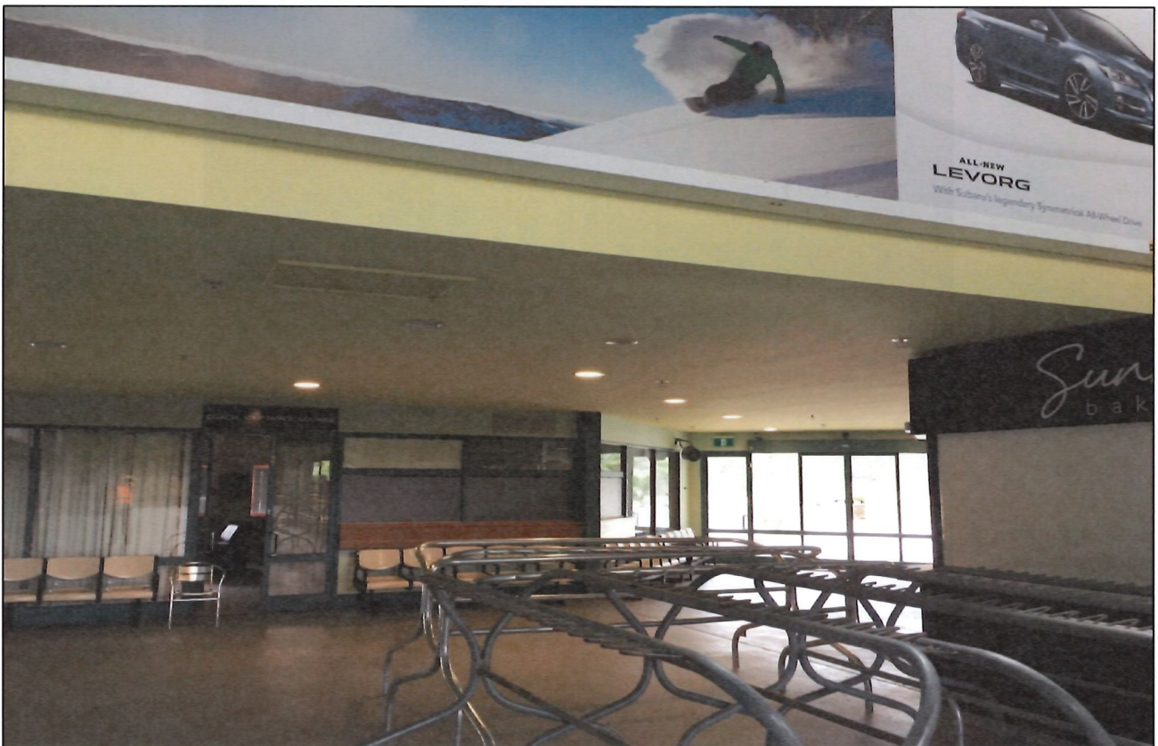
Figure 5: Proposed location of the Omni antennas above the coach driver lounge area.
